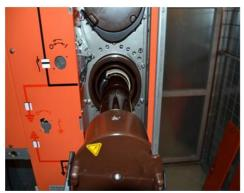
Fig. 1 Switchgear with HH fuse and TOC sensor adapted
